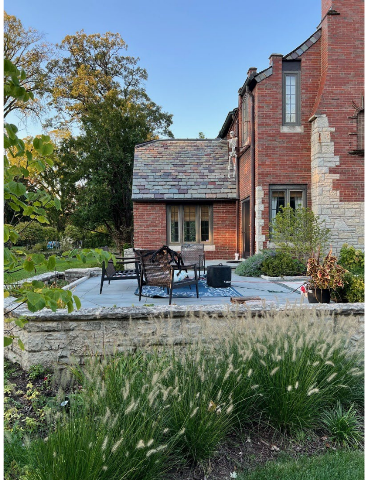
Existing patio at the Southwest corner of the house.
