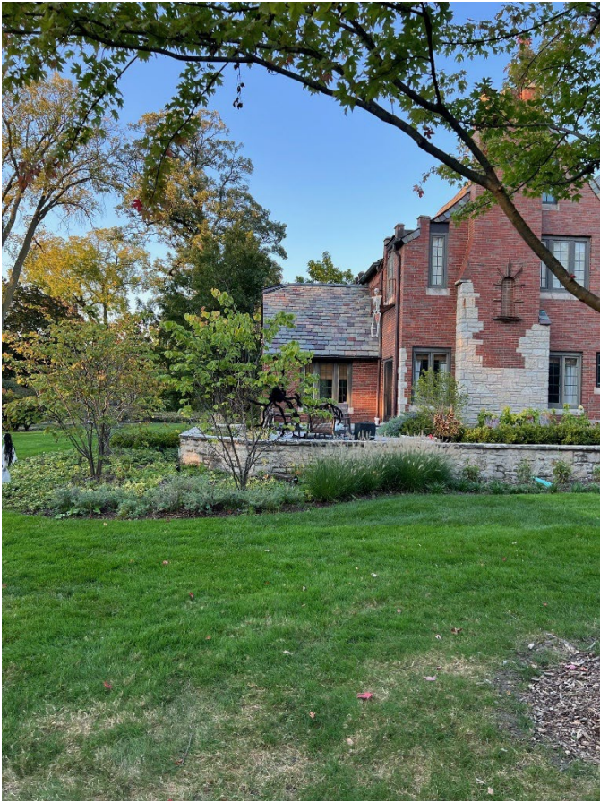
Southwest corner of the house. View from the south.
