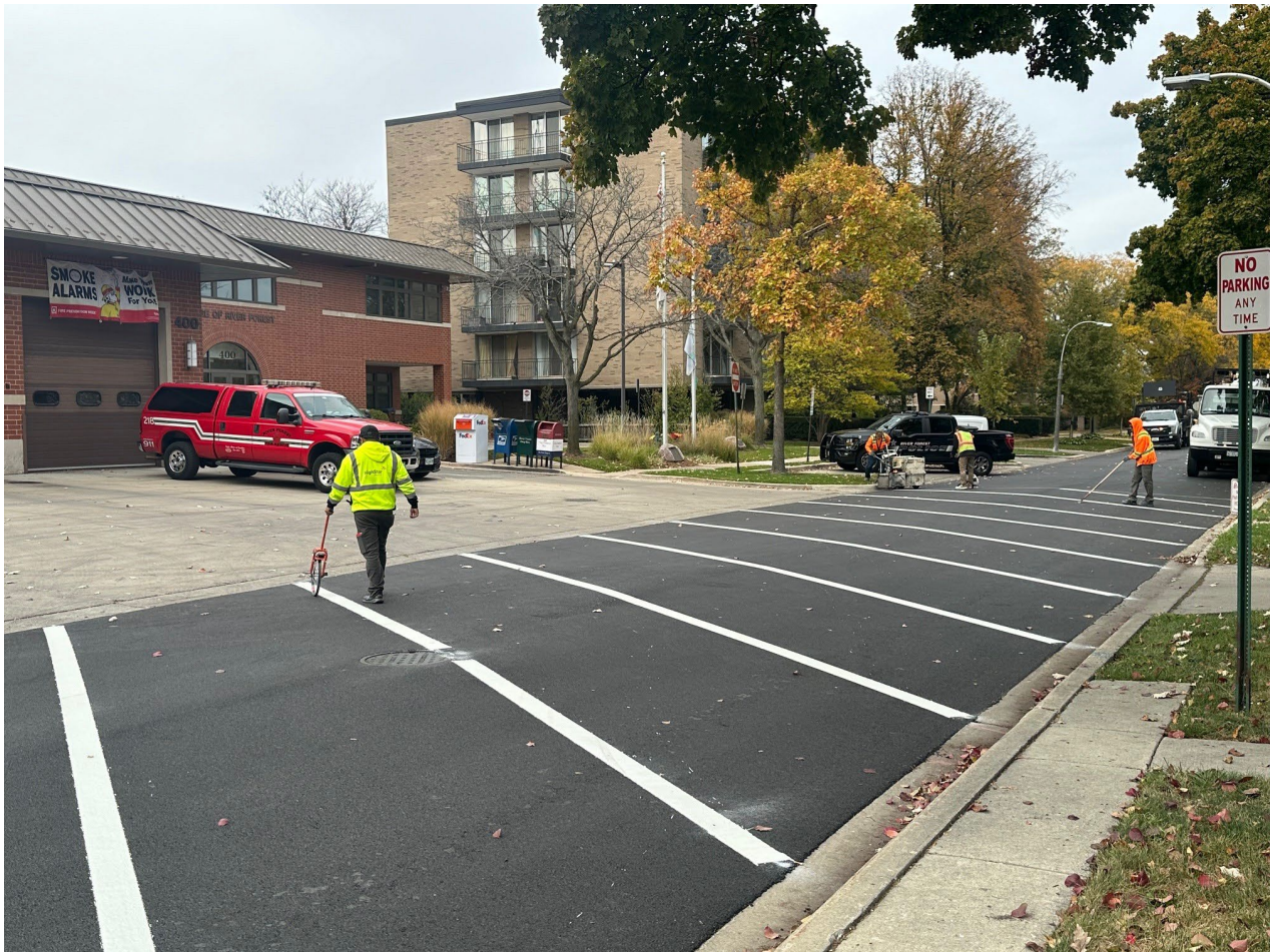
Village Thermoplastic Striping Project
