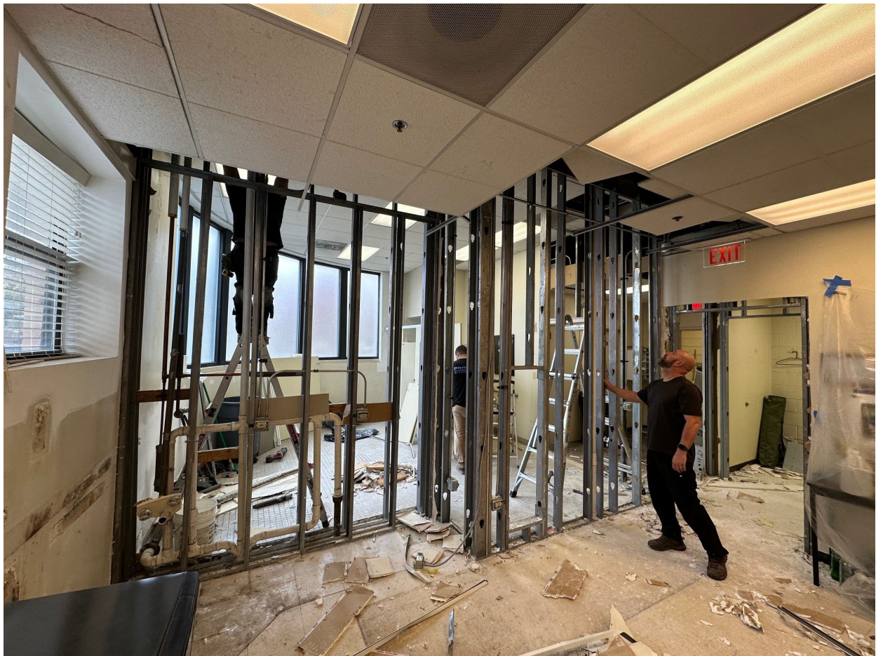
Public Works Interior Remodel In Progress
