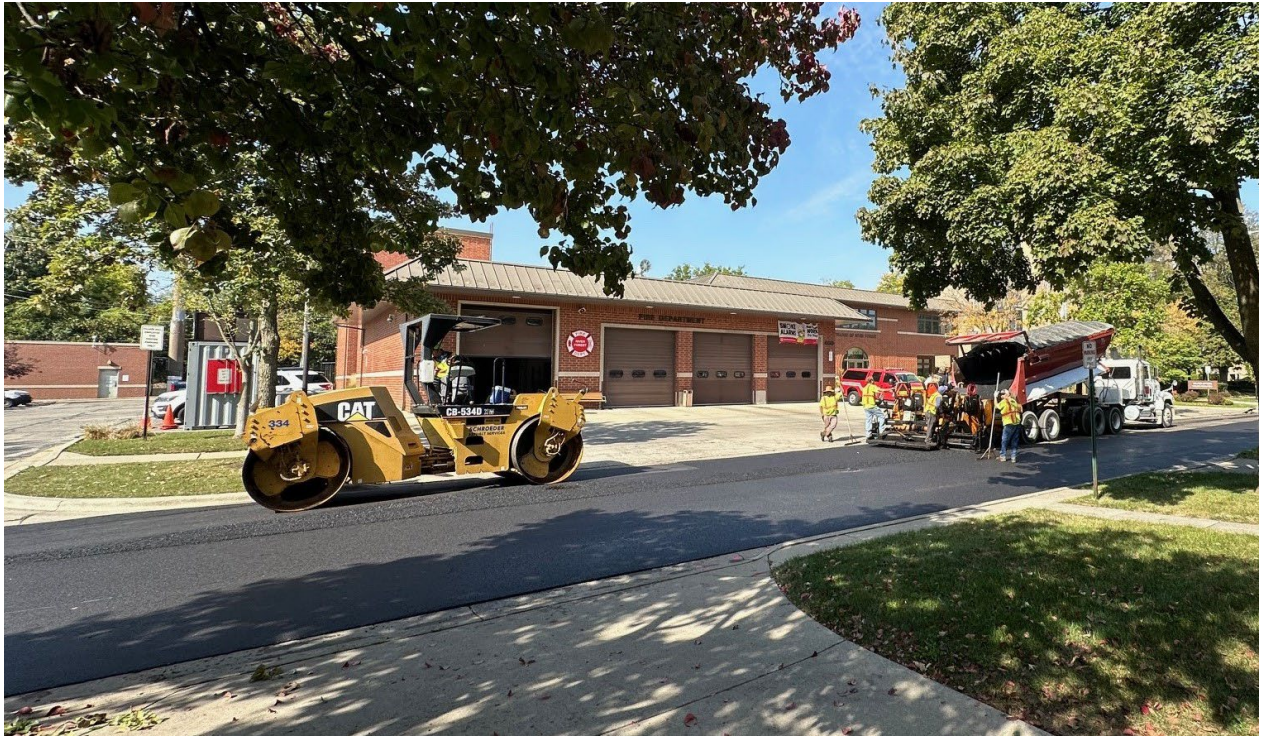
Village Street Patching Project
