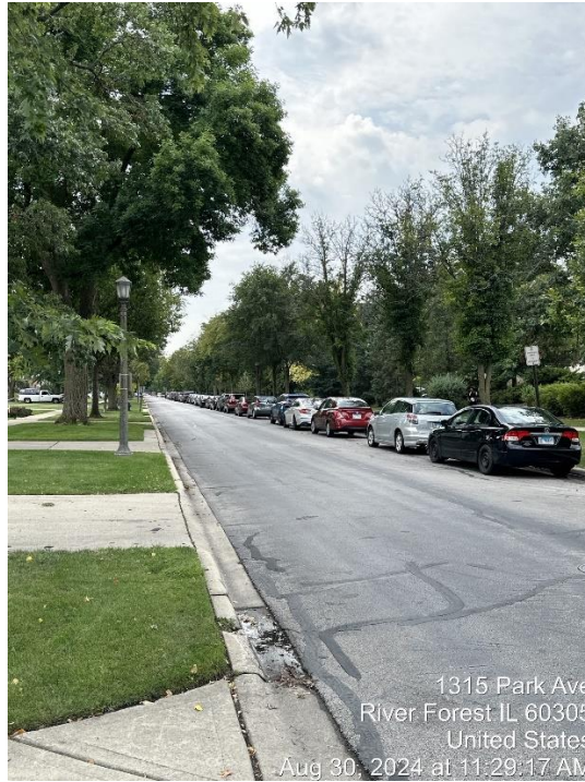
Along 1200-1300 Block of Park Avenue Facing South
