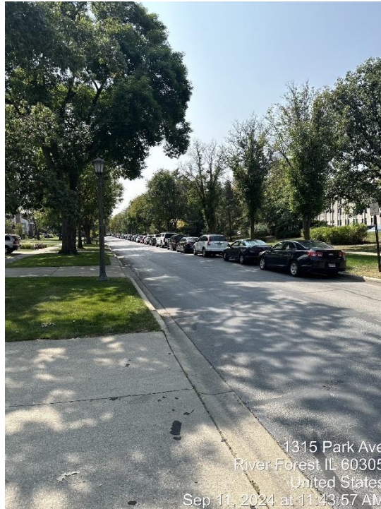
Along 1200-1300 Block of Park Avenue Facing South
