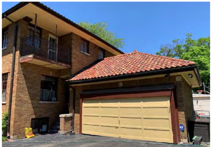
View of existing garage from south.
