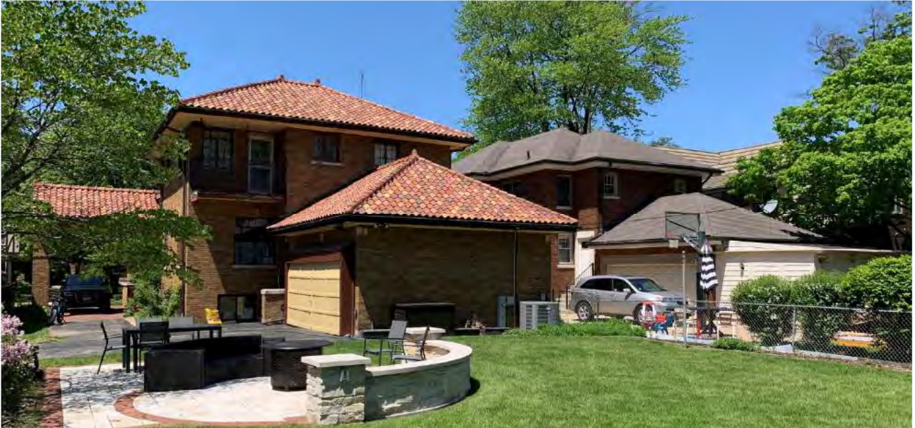
View from southeast of existing garage and house with neighbor to right.
