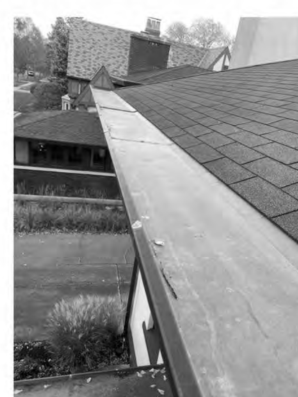
DETAIL OF EXIST GUTTER
