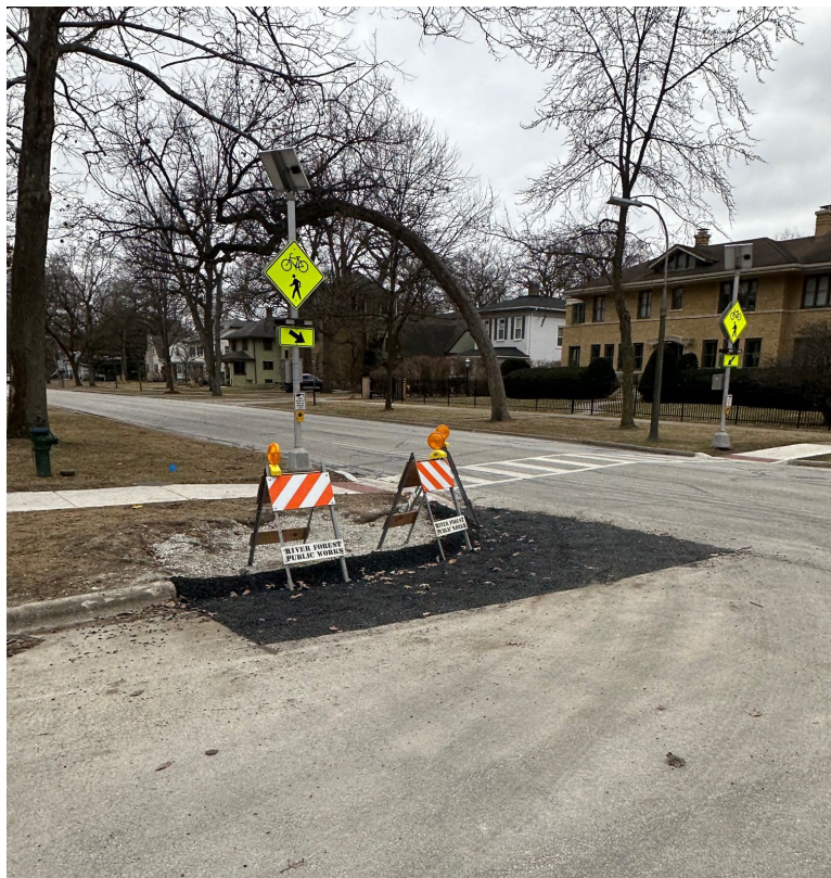
Temporary Pavement Patch
